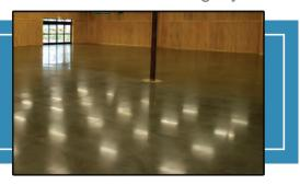
Kolour Dye™ is a translucent dye, formulated using very fine particles of color designed to penetrate and color interior cementitious surfaces. including polished concrete. Kolour Dve™ creates unique, color multi-colored translucent scheme. Kolour Dve™ is available in 19 standard colors but can be combined to create an unlimited color palate that creates a marble effect, when used properly. Create the look of a beautiful, custom acid stained floor in about 1/3 of the time.
