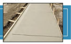
2500 LV UV 350 VOC is a UV resistant, low viscosity 25% solids solvent based acrylic copolymer curing and sealing compound, as well as a dust-proofer for concrete surfaces. 2500 LV UV 350 VOC offers improved resistance to rain, the sun, freezing temperatures, stains, and other pollutants that can often be hazardous to concrete. 2500 LV UV 350 VOC forms a moisture retentive film on freshly placed concrete.
